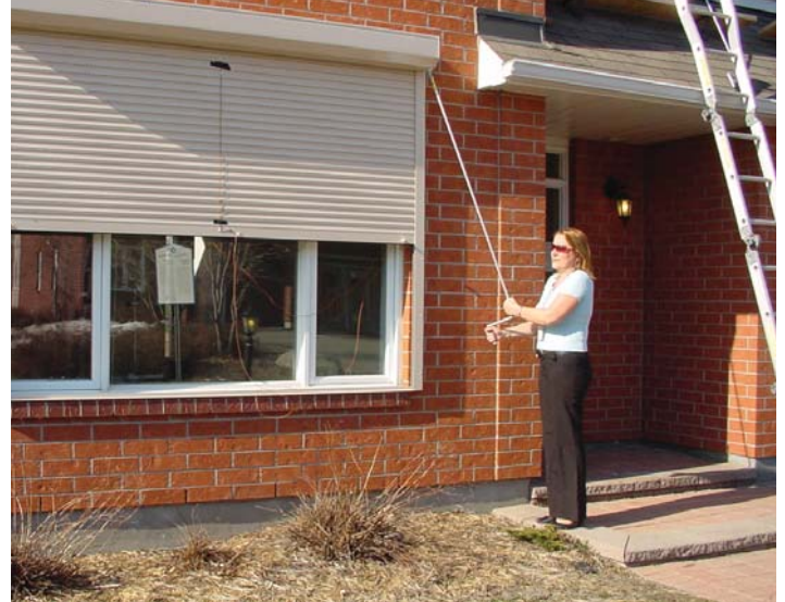
An experiment in the CCHT twin houses showed that exterior roll shutters provide substantial cooling energy savings on sunny summer days.
